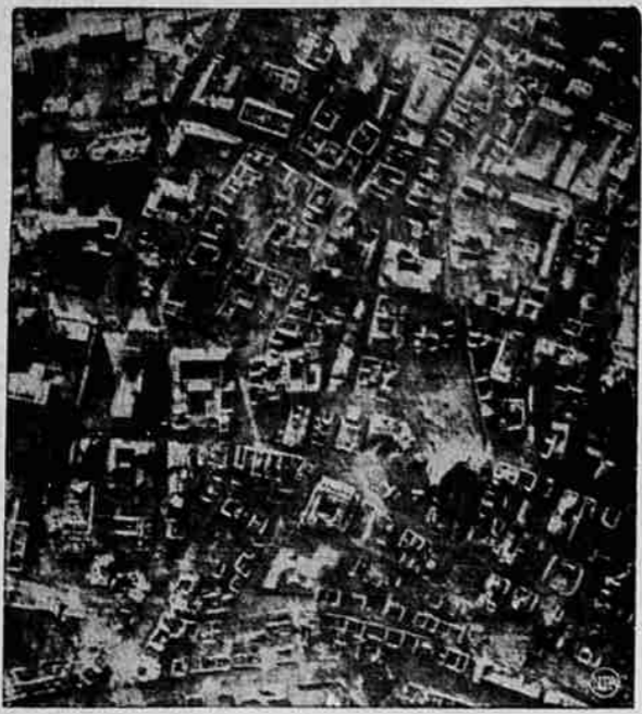
These blocks of burnt-out buildings, part of 140 devastated areas in Essen, are vivid evidence of the destruction wrought by RAF bombers in recent heavy raids on the German industrial city. Famous Krupp munitions works was partly destroyed here.
