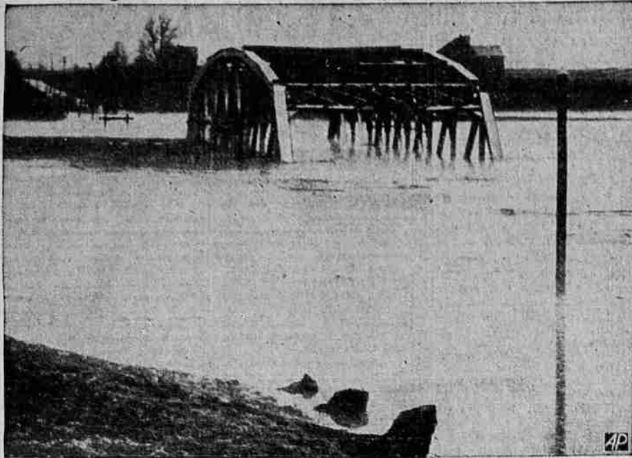
Rising waters flooded lowlands in Ohio, Pennsylvania and other states. This bridge on the Youngstown-Akron road, shows what happened when the New Berlin dam, near Youngstown, failed to release water as fast as it flowed into the reservoir.
