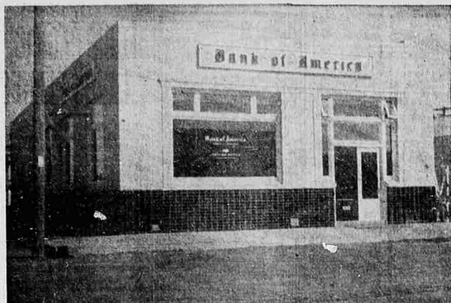
Monday, October 6, personnel of the Tulelake branch of the Bank of America will greet customers in this handsome new building, completed this week. Located on Main street, the bank offers all facilities to take care of the rapid growth of the community. In deference to war-time conditions, no formal opening is planned.
