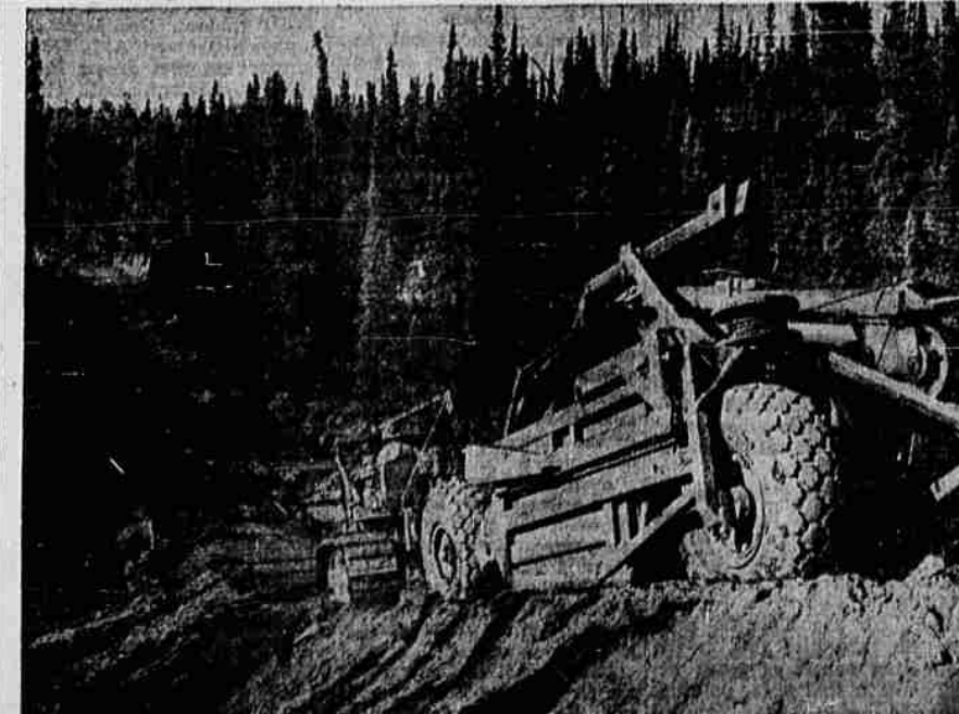
This mighty machine of peacetime, a tractor-drawn carry-all, helps build a wartime highway to Alaska through the forested Canadian wilderness. U. S. Army engineers constructing the road use this machine to move tons of earth from one section of the route to a hill.
