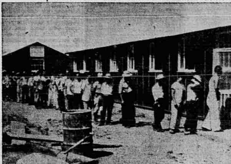
Japanese-Americans, evacuated from the Pacific coastal areas after the outbreak of war, set up their homes at Rohrer relocation center, McGehee, Ark., and these evacuees lined up for a meal in the mess hall. This advance contingent were volunteers for the task of preparing the center for other evacuees.
