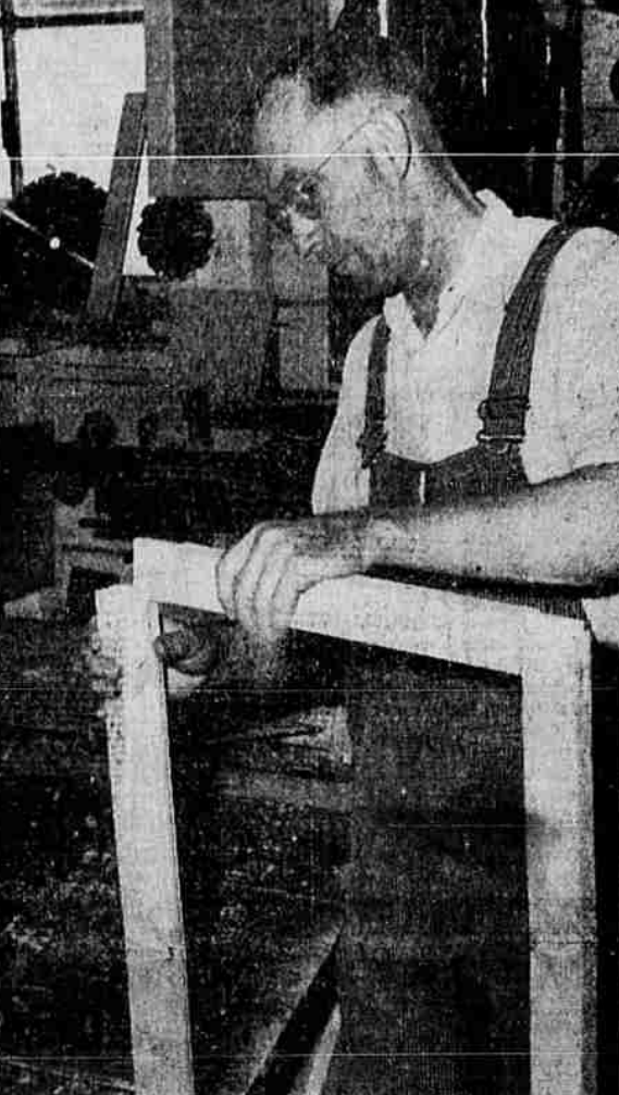
Picture shows E. S. Robinson of the Klamath Cabinet shop putting together one of the 14,000 sash which this local plant is producing for defense houses in Portland. Some 20,000 screens are also being produced here for pre-fabricated houses at an ordnance depot in Utah.
