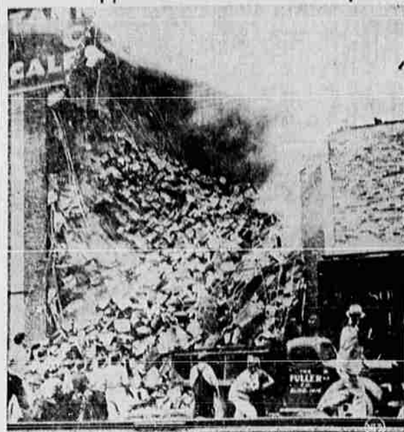
While rescuers worked to free 11 workmen believed trapped in the partial collapse of a Wauwatosa, Wis., brewery warehouse, another section of the building caved in. A photographer got this striking shot as wreckage, mingled with thousands of cases of beer, cascaded down to seal the trap on the workmen.
