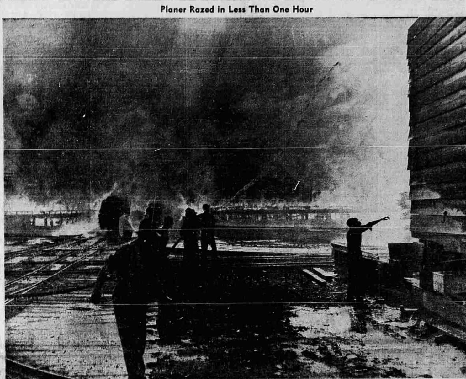
The entire Pelican Bay Lumber company planing mill and all its equipment was completely destroyed by racing flames which broke out at 5 o'clock Tuesday afternoon, leveling the old structure in less than an hour. The above picture, facing west, was taken after fire had razed the upper framework of the mill. The fire was quelled before it could take dry sheds and piled lumber surrounding the mill. Officials today said the mill would be rebuilt as soon as humanly possible.
