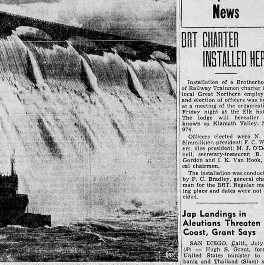
Beauty and utility are two qualities of Grand Coulee Dam, in eastern Washington. More than 6000 tons of water spill over this dam every second in this spectacular man-made waterfall twice as high as Niagara. Three 150,000-horsepower turbines have harnessed a portion of the Columbia River's flow to supply a large block of power to essential war industries.
