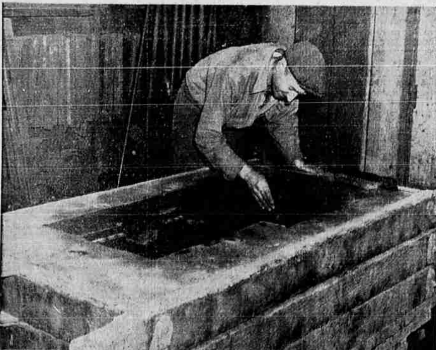
HANDLE WITH CARE —Ivan Lehrman in the foundry puts the finishing touches on a mold preparatory to its being poured full of molten iron. Inside is an air space made from Hayden's pattern and surrounded by sand.
