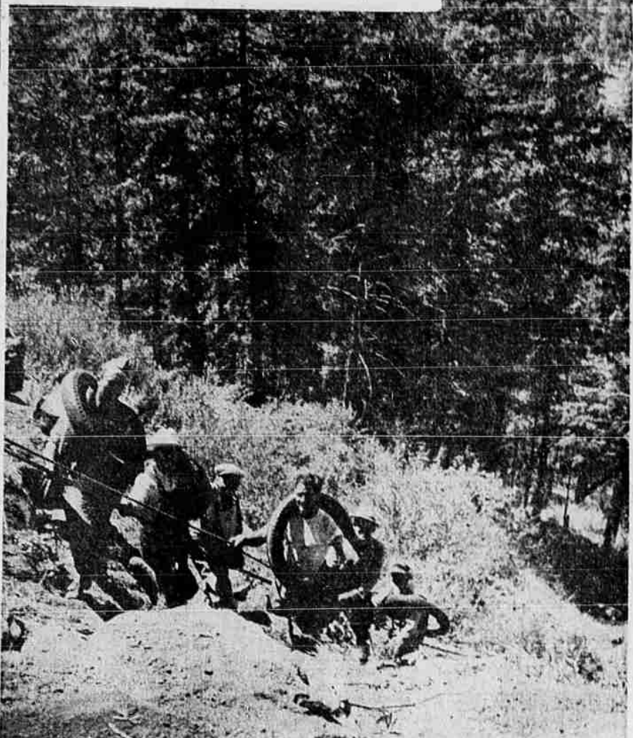
BRINGING OUT THE RUBBER —It was tough going but it was worth it when a group of Klamath service station and oil men recovered a ton of old rubber from the Klamath river canyon Thursday. Ropes were strung down the canyon wall to help bring up the tires. Those in the party were Marshall Cornett, J. H. Morgan, C. E. Newcom, Cal Frei, Kenneth Weber, Ray Broilier, Harry Coleman, Loyce Mitchell, Robert Fulton and John Schubert. They worked all afternoon and well into the night on the job, bringing up the rubber for the defense scrap pile.
