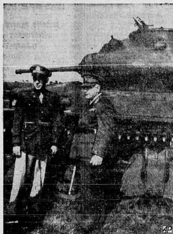
General Richard K. Sutherland (left), of the U. S. army, and Colonel W. D. Watson, Australian army tank designer, stood before one of the heavy Australian-built cruiser tanks at a display of equipment given by the Australians for newly arrived American soldiers.
