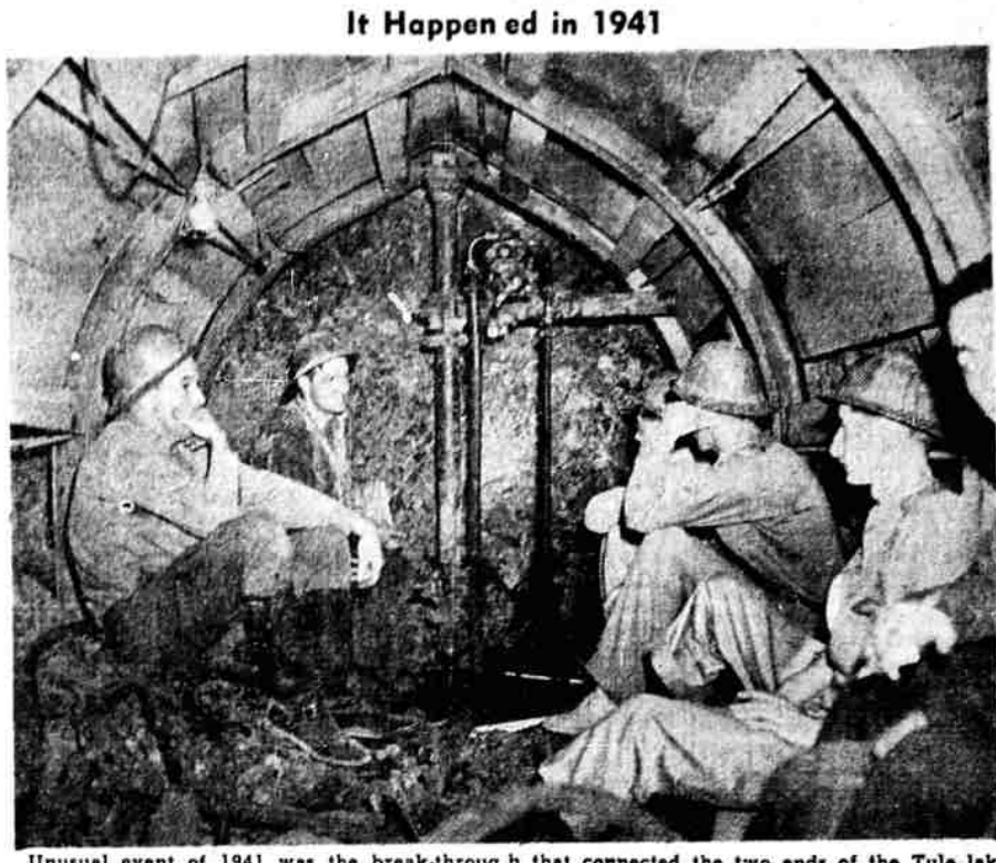
Unusual event of 1941 was the break-through that connected the two ends of the Tule Lake-Lower Klamath lake tunnel. Picture shows crew waiting for the drills on the other side of the wall to bore the first hole.
