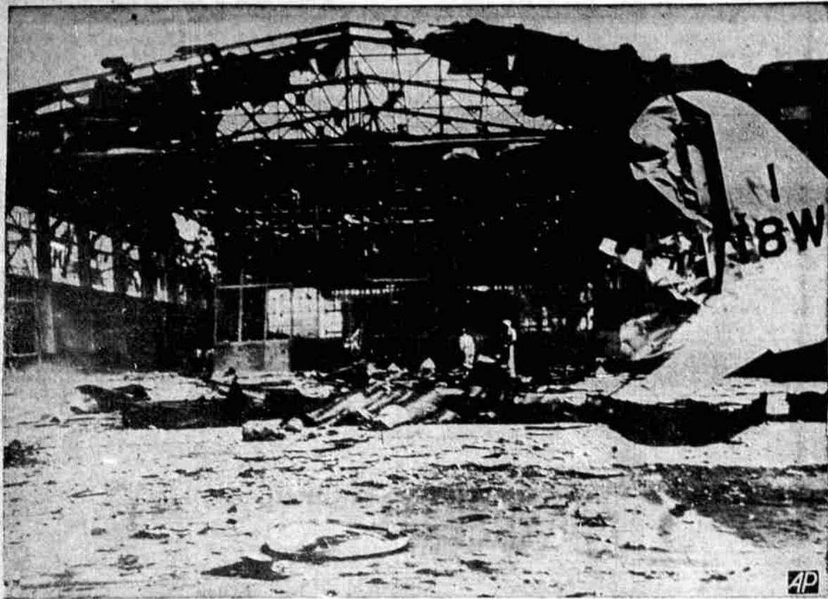
WINGED DESTRUCTION HITS HICKAM FIELD —A major object of the Japanese bombing raid on Honolulu. Hickam field was littered with wreckage. This is one of the first pictures of the destruction released by the army and shows one of the damaged hangars.
