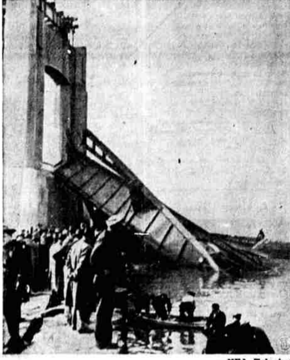
When three huge spans of the world's largest girder bridge, being constructed over the Connecticut river at Hartford, Conn., collapsed and plunged 150 feet into the water, 10 workers were killed, four missing and at least 17 others injured. Here's the shore end of the $4,400,000 bridge after it fell.
