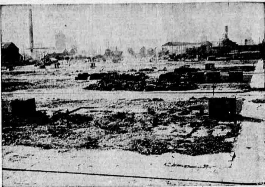
Four months' clearing labor completes work of German bombs in the dockland section of London, leaving a great area bare except for the little surface shelters that stood up under the attacks.
