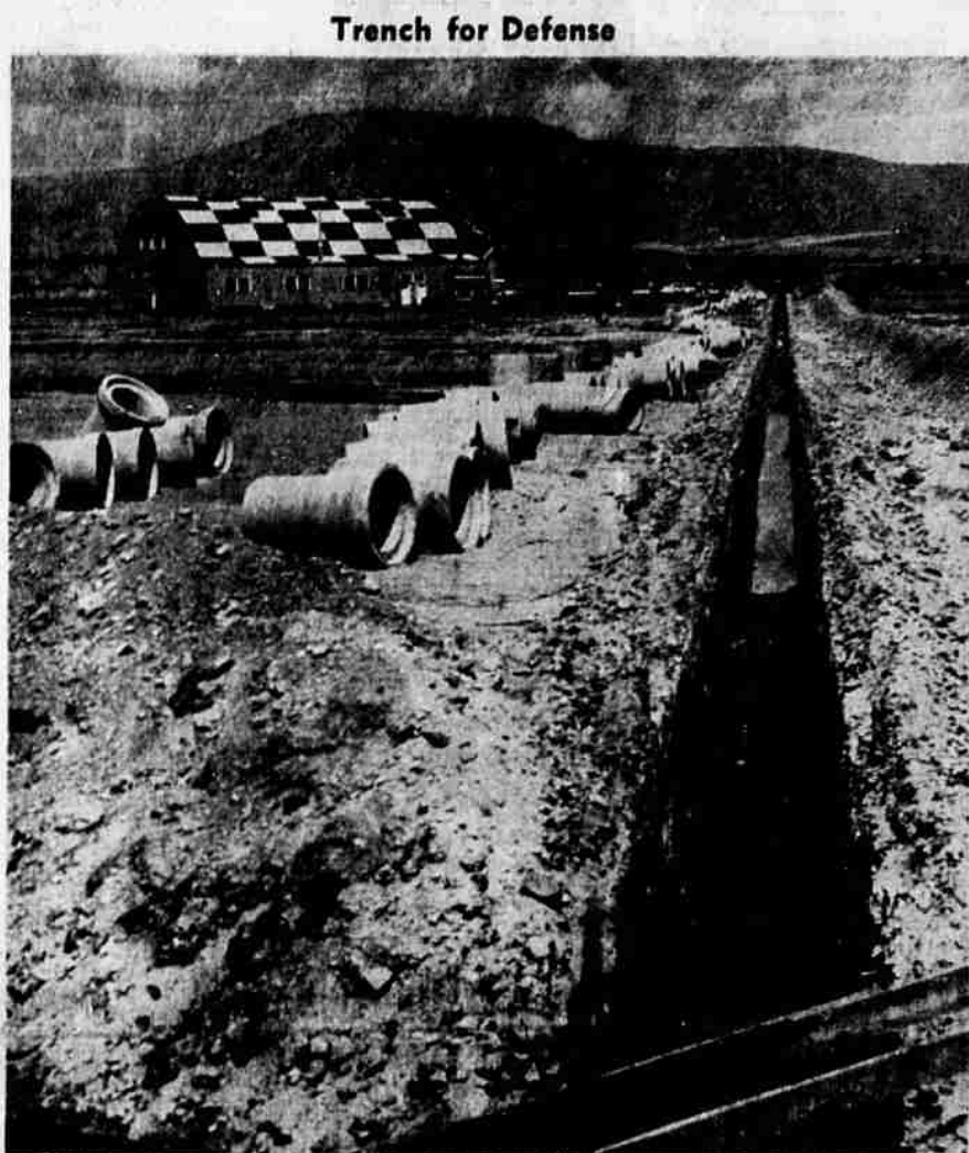
Trench for Defense
