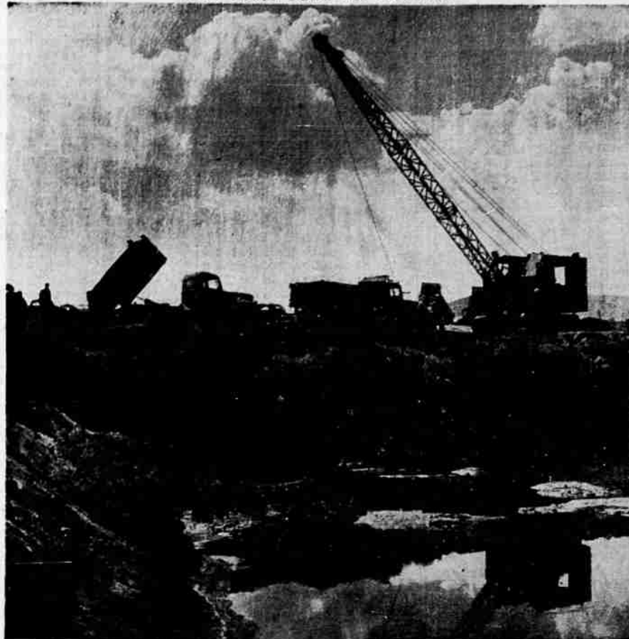
Runway beds for the $319,000 Klamath Falls municipal airport defense project are being constructed from sand taken from what engineers believe is the old bed of Lost River at the airport's south end. Above, a crane is loading the sand onto trucks.
