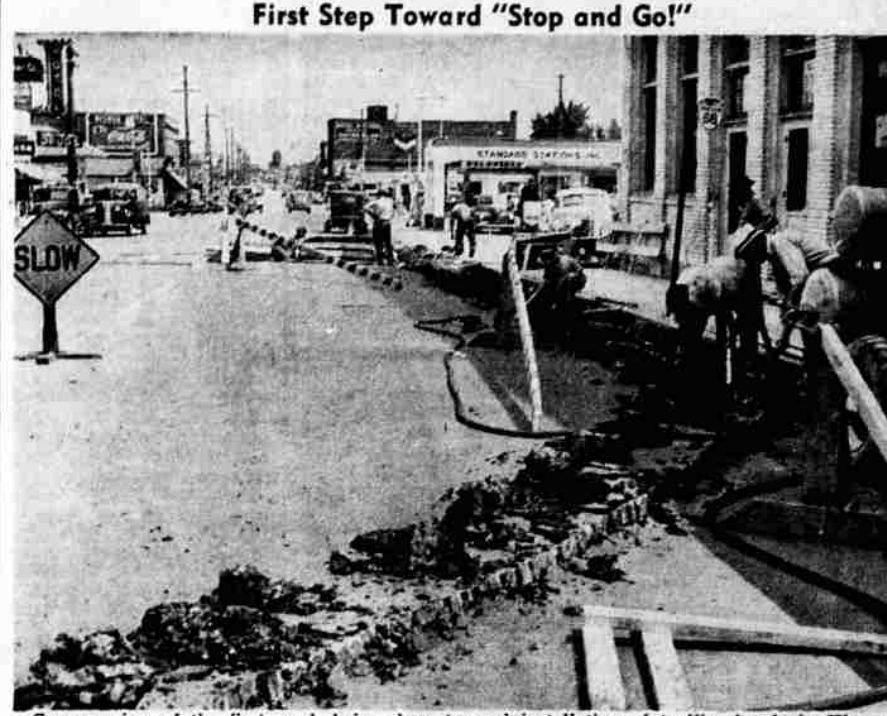
Camera view of the first work being done toward installation of traffic signals in Klamath Falls. South Sixth from Main to Klamath presented this untidy but gratifying scene.
