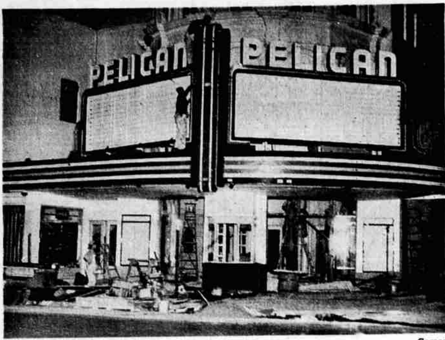
A new face, which cost Klamath Theatres, Inc., just $25,000 was being given the Pelican theatre which opens Friday afternoon after being "dark" for the past few weeks. Workmen were putting the last touches to the huge new marquee when this picture was taken.
