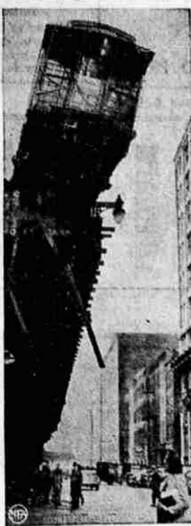
Chicago elevated train crashes through guard rail at dead end station and dangles over street. Cause: failing brakes. Result: no injuries to passengers.
