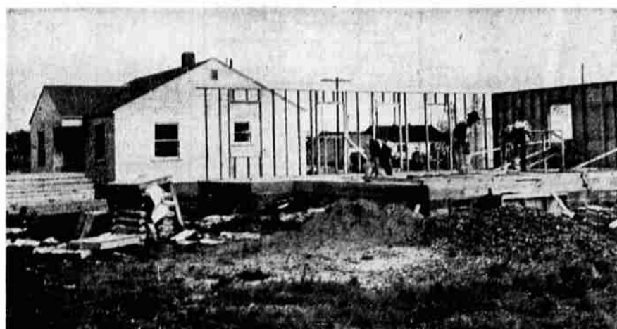
Largest number of permits last week went to Gerard Klinkhammer, contractor, who has a number of small homes under construction in the city limits. Above, two of the houses now being built on Wantland avenue. Mills addition.
