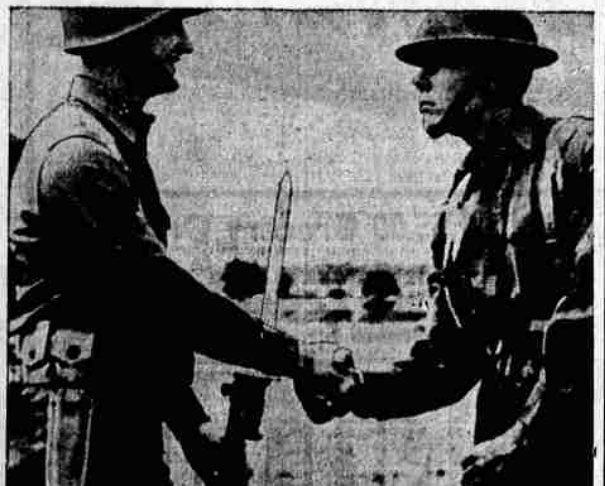
A new steel helmet, left, offering better protection than the old type, right, is under exhaustive test by the Infantry Board at Ft. Benning, Ga. Designed to protect neck and side of head, it has a fiber lining, which, worn alone, may replace the present overseas cap.
