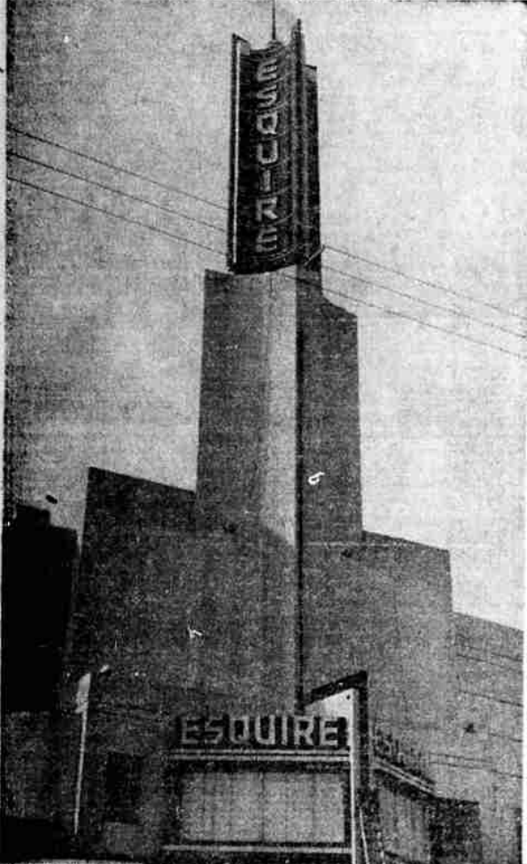
CONSTRUCTION —Construction was active through the year, a top-notch item being the handsome Esquire theatre at Seventh and Pine streets. Picture shows the Esquire sign, new feature of the local skyline. George Mann, owner of the Esquire, is also building a theatre on South Sixth street.
