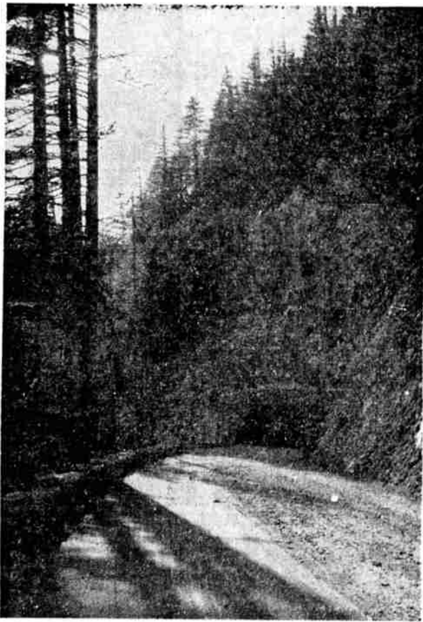
NEW HIGHWAY —Big event of the year for the Klamath country and coast travel in general was the opening of the new Willamette highway. This picture shows the highway at the entrance of the Salt creek tunnel.
