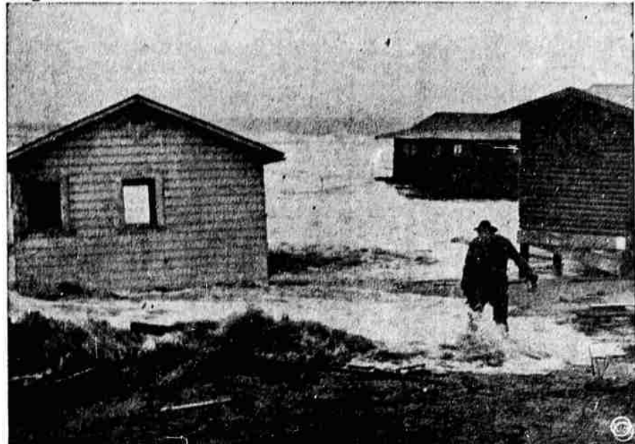
Huge breakers curl around, undermine and toppled cottages at Stinson Beach, near San Francisco, during high tide and heavy winds that caused extensive damage.
