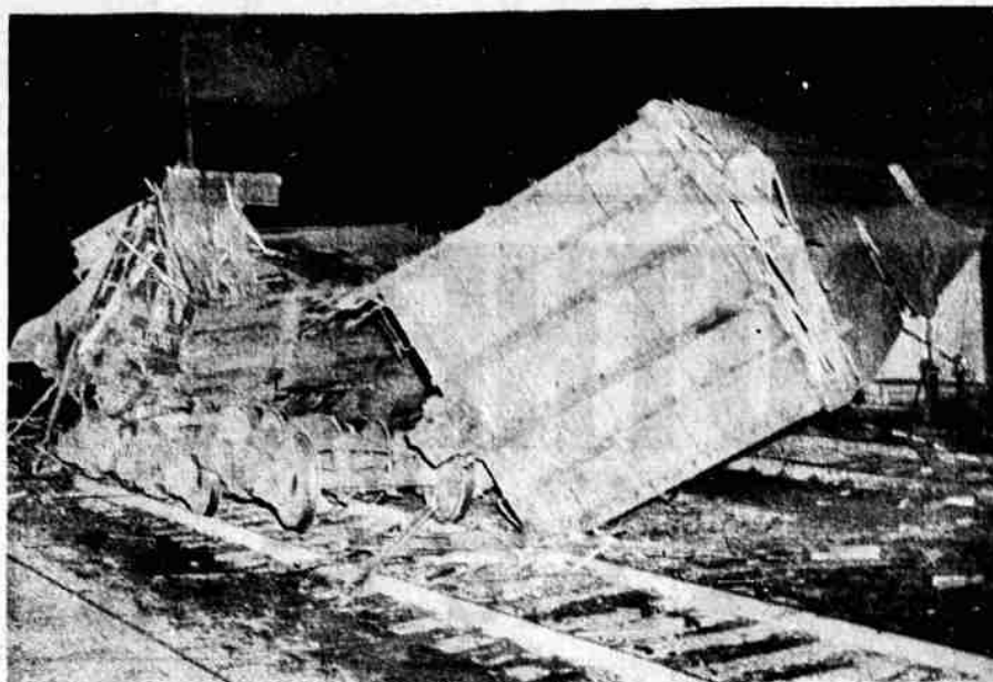
The demolished caboose (left) and a boxcar draped over a switchhouse are shown above as they appeared after a collision between a locomotive and the rear end of a freight train in the Klamath Falls yards Thursday night.
