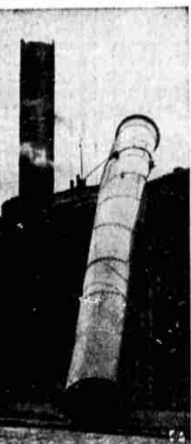
DOWN DRAFT—Only half a chimney stands where once a whole one thrust up into the sky. This is what the wind did to a wool scouring plant stack at Philadelphia.
