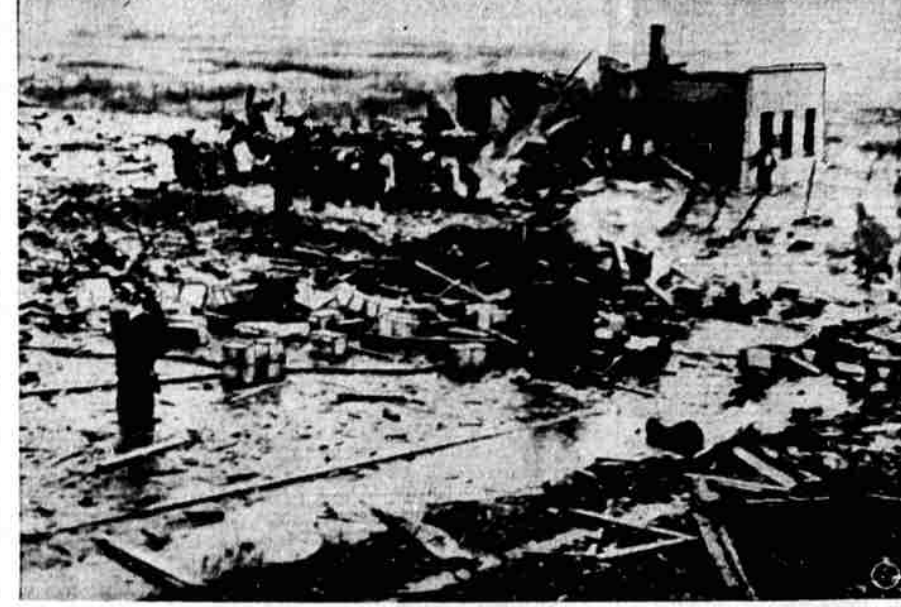
At least eight persons were killed and 26 injured when an explosion raged the United Railways and Signal company's plant at Woodbridge, N. J., above. Shortly before, blasts in two Pennsylvania powder plants killed at least six other persons. Federal bureau of investigation launched an investigation of the three explosions.
