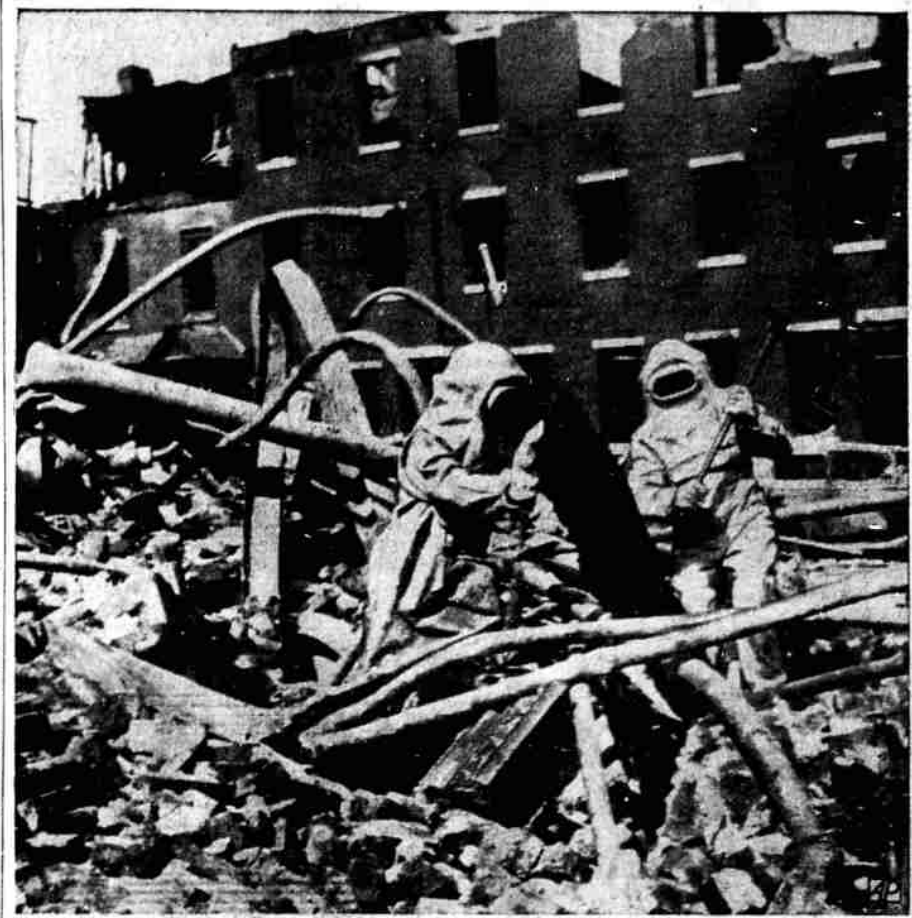
Resembling mythical "men of Mars" in their asbestos suits, these firemen are digging into the fire-twisted wreckage of the R. M. Hollingshead plant at Camden, N. J., in search of possible victims of a $2,000,000 disaster.
