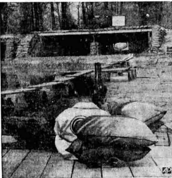
TEST OF PLANE TANK—Taking a hint from the European war, U. S. military experts now see the need of a fire-proof and leakage-proof gasoline tank for airplanes, and here's how a test was recently staged at the Glenn Martin plant in Baltimore. Above, a runner fires .30 caliber tracer machine gun bullets at an old style gas tank. See it in the sandbagged dugout.
