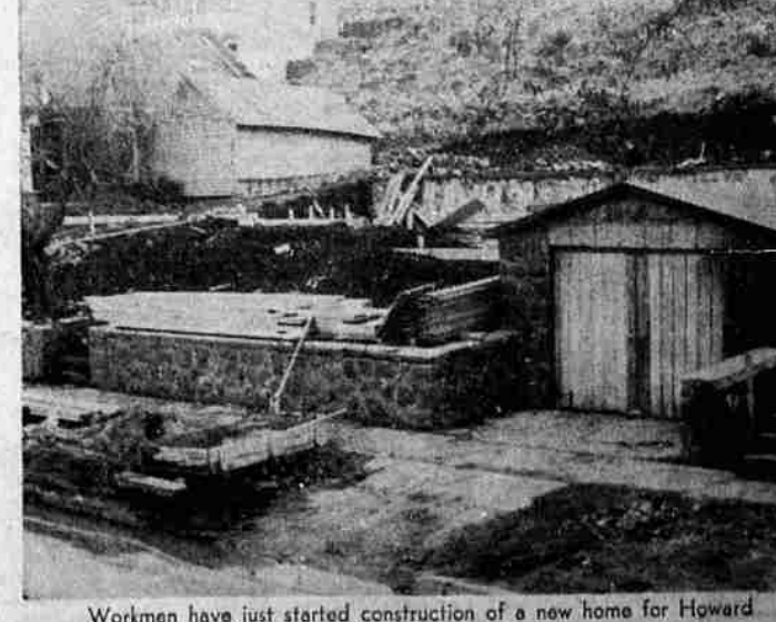
Workmen have just started construction of a new home for Howard Pernell on this hillside site on Riverside avenue.
