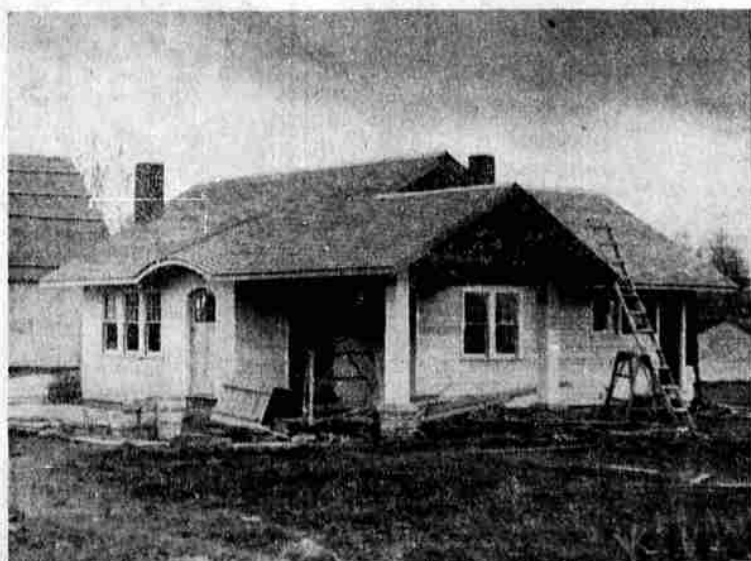
William Tiller is constructing this new home on Millers lane.
