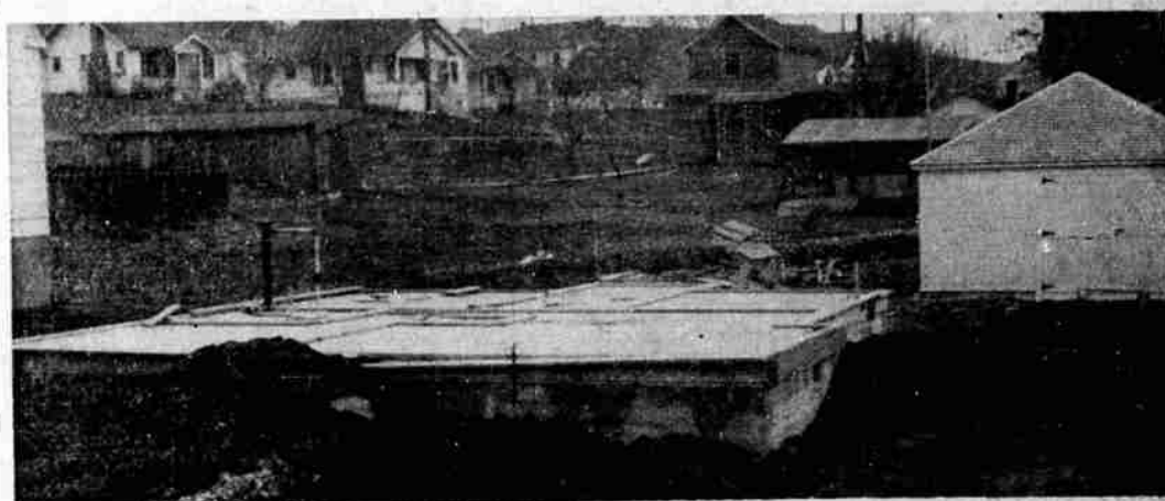
First steps in the construction of a new home for G. Gardner on Portland street are shown in the above picture.
