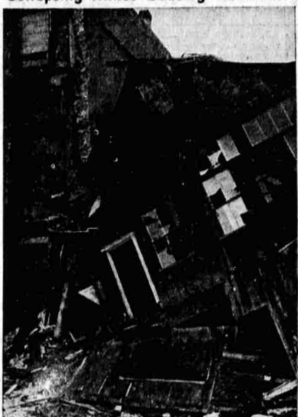
Collapsing mining tunnels and shafts that once produced a billion in gold and silver at Virginia City, Nev., now are causing the earth to settle and fall of many landmarks. Here, one of the town's oldest structures collapses after the cornice from an adjoining building broke off, dropping tons of brick and mortar.
