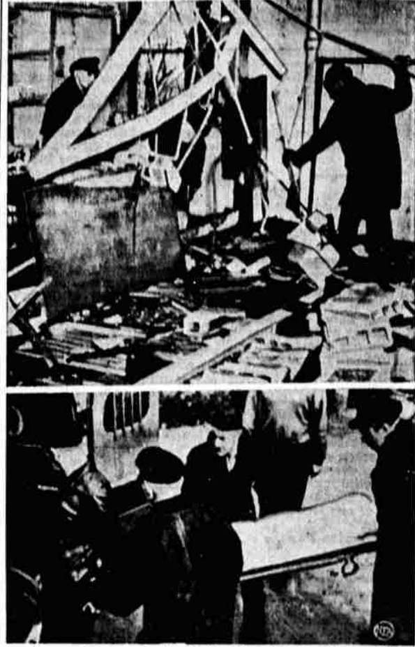
Above, interior of the Booth Memorial hospital at Cleveland, Ohio, where a gas explosion wrecked the laboratory, shattered 40 windows and injured seven women members of the staff. Lower, police remove one of the victims of the blast.
