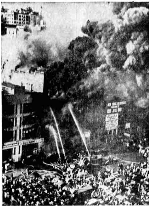
One fireman was dead and six injured when the roof collapsed in this $400,000 fire which struck a five-story Los Angeles factory building. The fire was reported caused by Samuel Trevor, who took his dog for a walk and left a hot plate turned on in his second-floor shop. This is a general view of the blaze.
