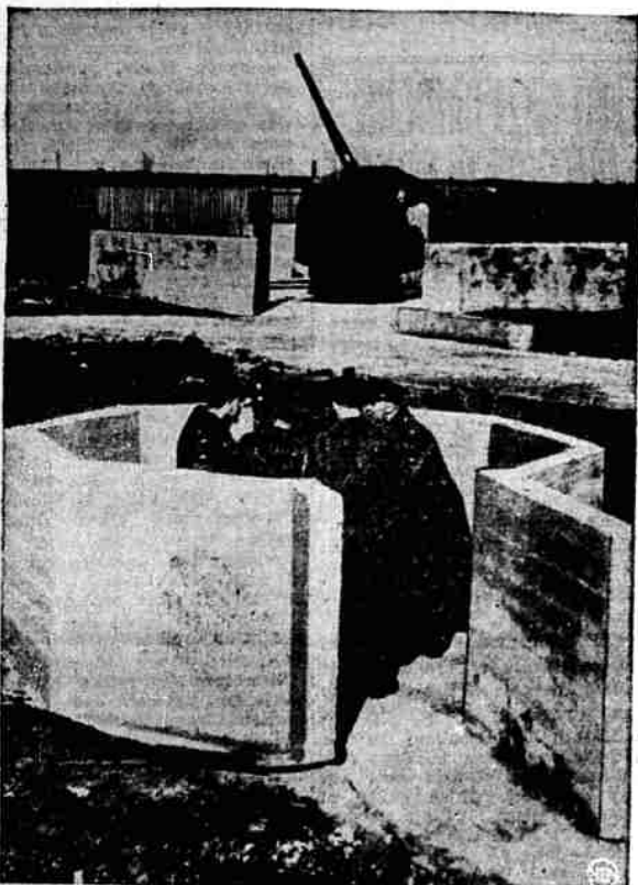
Its air raid defense stepped up by Nazi bombing raids in Scotland, Britain counts heavily on a new 4.5-inch anti-aircraft gun, background, to repel enemy planes. A gun crew in reinforced concrete emplacement, foreground, operates the "predictor" that locates raiding planes, supplies range for guns. These new guns have been set up in the London area.
