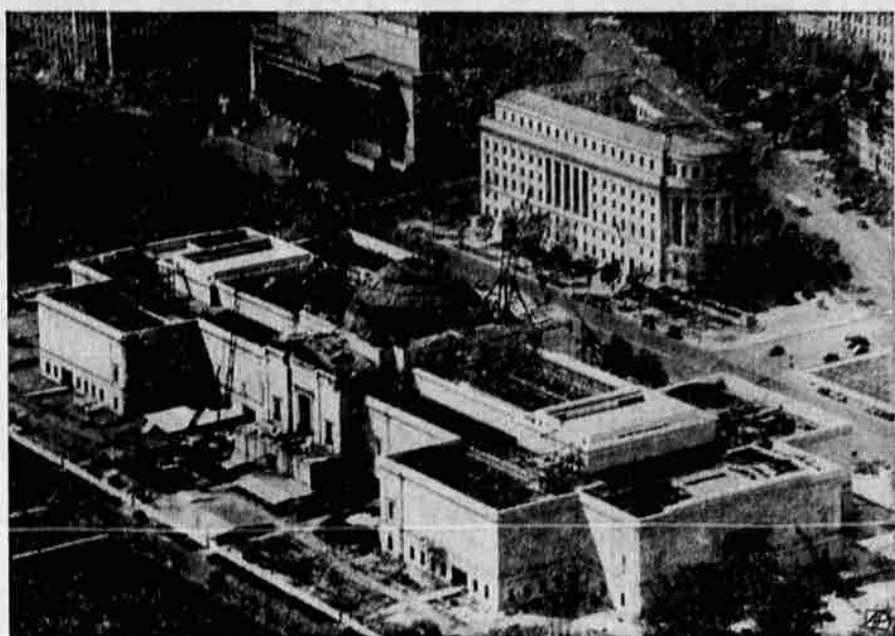
NATION'S NEW ART GALLERY—Here's a view of progress on the national art gallery in Washington, D. C. In rear are the apex, or trades, building and the archives building (left).
