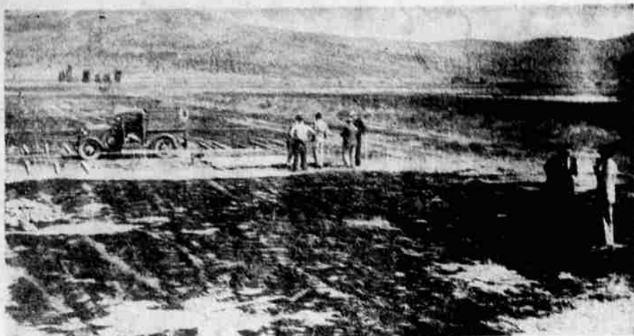
Picture shows work going ahead on a mobile camp for potato pickers being established at Merrill.
