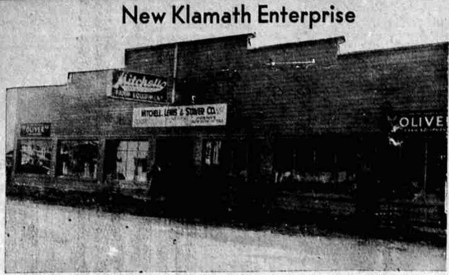
View of the Mitchell, Lewis and Staver farm implement establishment on South Sixth street. This is a new business in Klamath Falls, located in a new building adjoining the Klamath Valley Lumber company plant on South Sixth street. (Herald-News Photo-engraving).
