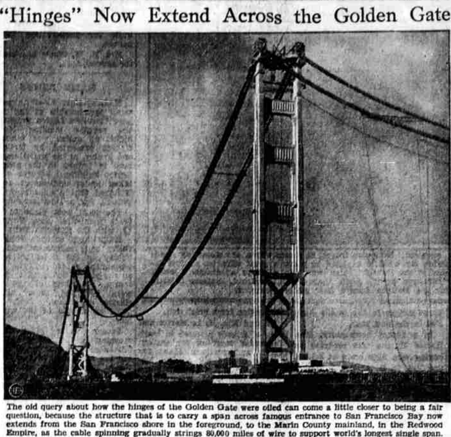
The old query about how the hinges of the Golden Gate were oiled can come a little closer to being a fair question, because the structure that is to carry a span across famous entrance to San Francisco Bay now extends from the San Francisco shore in the foreground, to the Marin County mainland, in the Redwood Empire, as the cable spinning gradually strings 80,000 miles of wire to support world's longest single span.
