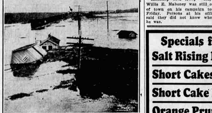
Clinton Junction, Okla., is only a speck on the map at its best, but even that speck was hard to find after six feet of water rushed over the town when the Washita river went on a rampage as shown here. The rail station kept its equilibrium, but other buildings toppled before the torrents. The flood took more than a dozen lives down stream.
