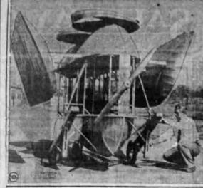
"This weird device is a cross between an airplane and a helicopter and is called a "mobilopter." Harry Cordy of El Monte, Calif., seen at its side, is its designer. The wings fold in and flatten out as the ship rises and descends. Those air screw discs on the top pull it upward, and the propeller pulls it forward. Cordy expects to test
