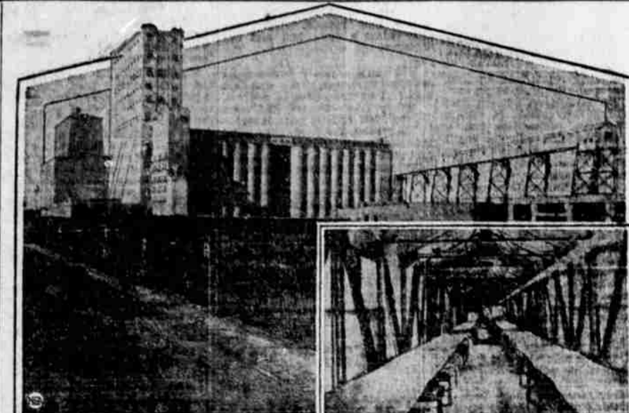
This recently completed elevator at Galveston, Texas, has a capacity for 6,000,000 bushels of grain. At right are two of the 42-inch belts which convey the grain to and from storing bins.
