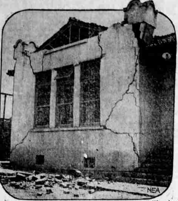
Here's what happened to a schoolhouse near Whittier, Calif., when a slight earthquake jolted the southern portion of the state the other day. No serious damage was done, but cracked walls, broken windows and loosened roofs gave citizens a number of thrills.
