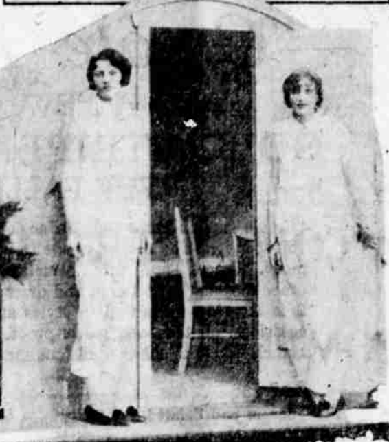
The "desert submarine" . . . is made of wood, sheet metal and flannel . . . water running over it evaporates, reduces the temperature 40 or 50 degrees.
