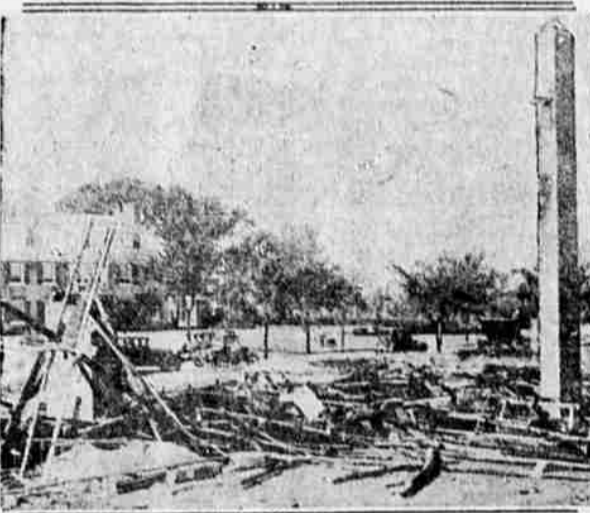
The chimney was all that remained of a nearly completed $40,000 home in Kansas City after a terrific and mysterious explosion.
