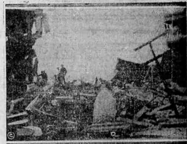
Once this building covered a whole block in Santa Barbara. Today it is a demolished structure, shaken to the ground by the earthquake last Monday.
