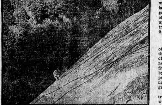
The almost perpendicular cliff looking from the top and showing how the workmen are suspended high above the plain.
