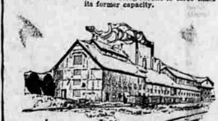
Plant No. 14—Gypsum Oregon. Another Certain-teed Acme plant producing gypsum cement plaster and gypsum blocks. The lightness, fire-proof qualities and speed with which walls can be constructed with gypsum blocks are causing them rapidly to displace other methods.
