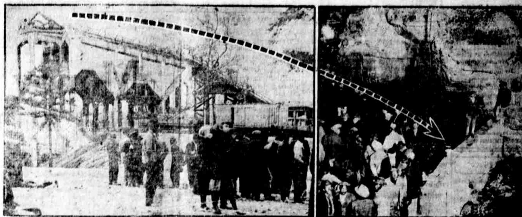
Eighty-four miners were killed by a freak explosion in the Dolomite coal mine, Birmingham, Ala. The dotted line shows the course of the dump cars which broke away, tore down the tippie and, after going down on the 800-foot incline, crashed into the yard below. Great clouds of coal dust arose. A high-tension electric cable severed at the crash and ignited the dust. In the terrific explosion, 40 men were killed outright at the foot of the tippie. Deadly after-damp accounted for the remainder of the victims.
