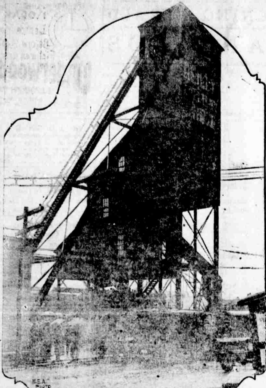
Waiting for news from the miners buried in the Spangler, Pa., mine disaster, in which more than a hundred lives were lost. Picture shows Reilly colliery No. 1, where the accident occurred, with anxious crowds gathered waiting first news. Notice the ambulances awaiting the injured.
