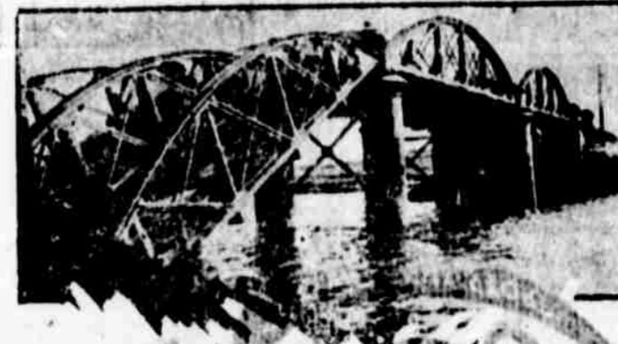
The Fort Bridge on the C. & W. railway between Queenstown and Cork, which was wrecked by Irish Irreguiars to halt advance of Free State troops.
